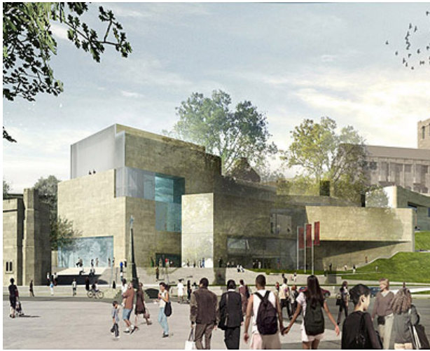
At Bangor University in Wales, construction is underway on the Grimshaw -designed Arts and Innovation Centre, also known as the Pontio project. Image: Grimshaw Extra Large Image
