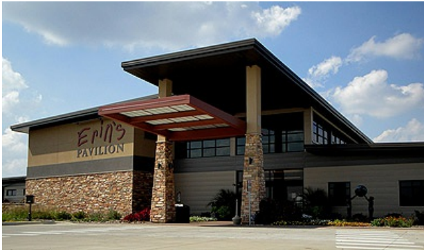
Erin's Pavilion at Edwin Watts Southwind Park in Springfield, Illinois, recently received LEED Platinum certification. Photo: Courtesy Walton Group Extra Large Image
