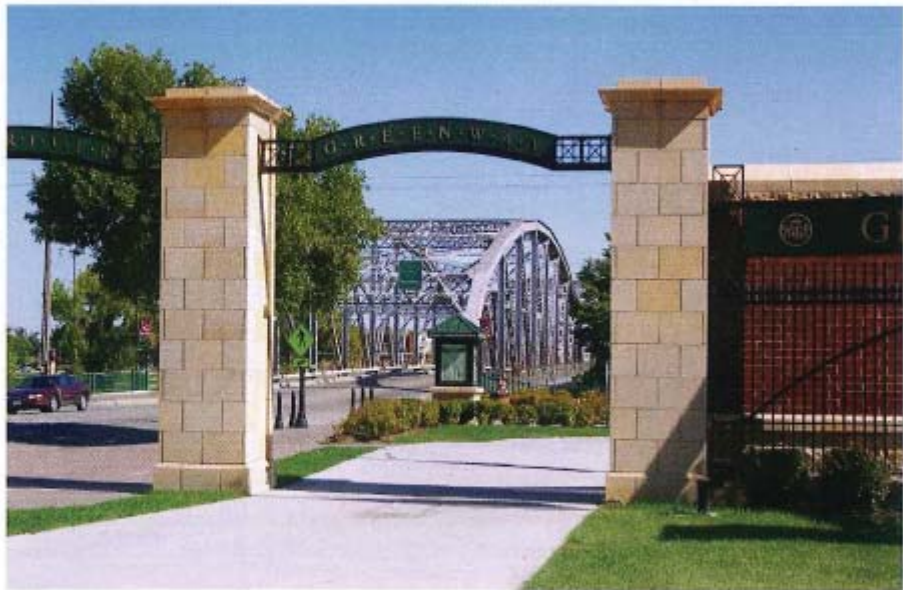
Though it might seem counterintuitive, the designers felt that the flood protection should be permeable, allowing, for instance, connection between downtown Grand Forks and the river. This is not, however, the norm with flood protection projects—even those being built today.
